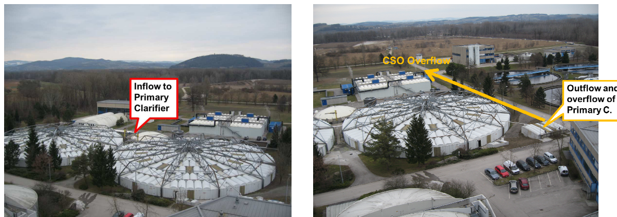
Figure 4: Photos of primary clarifiers indication inflow, overflow and outflow situation
